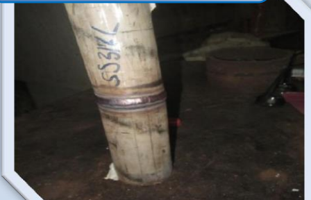
Hard Stamped after Welding Completion
